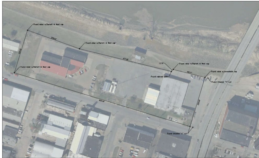
Figure 11. Topeka Metro Operations & Administration and Maintenance Facilities Ariel View Facing North 10
