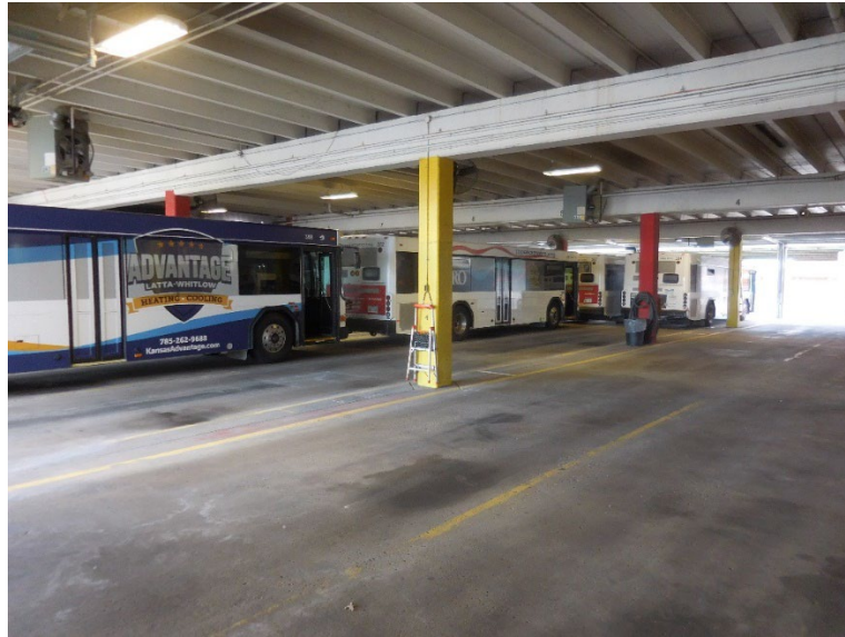
Figure 12. Interior Photo of the garage area at the Administration & Operations Facility
